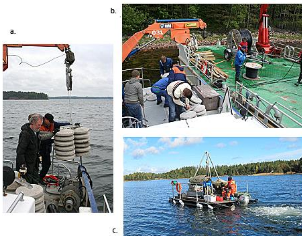
Figure 3-4. Set-up and removing of Mixox pumps in Sandöfjärden: a) anchoring (2009) b) cabling and anchoring (2009) c) removing (2011).
